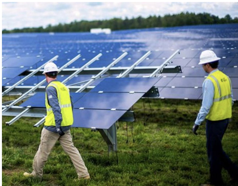
Duke Energy solar generation construction | Duke Energy
