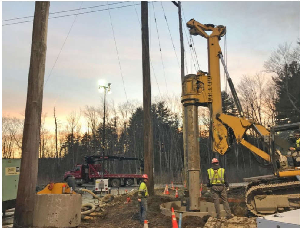
345-kV transmission line foundations | Michels Power
