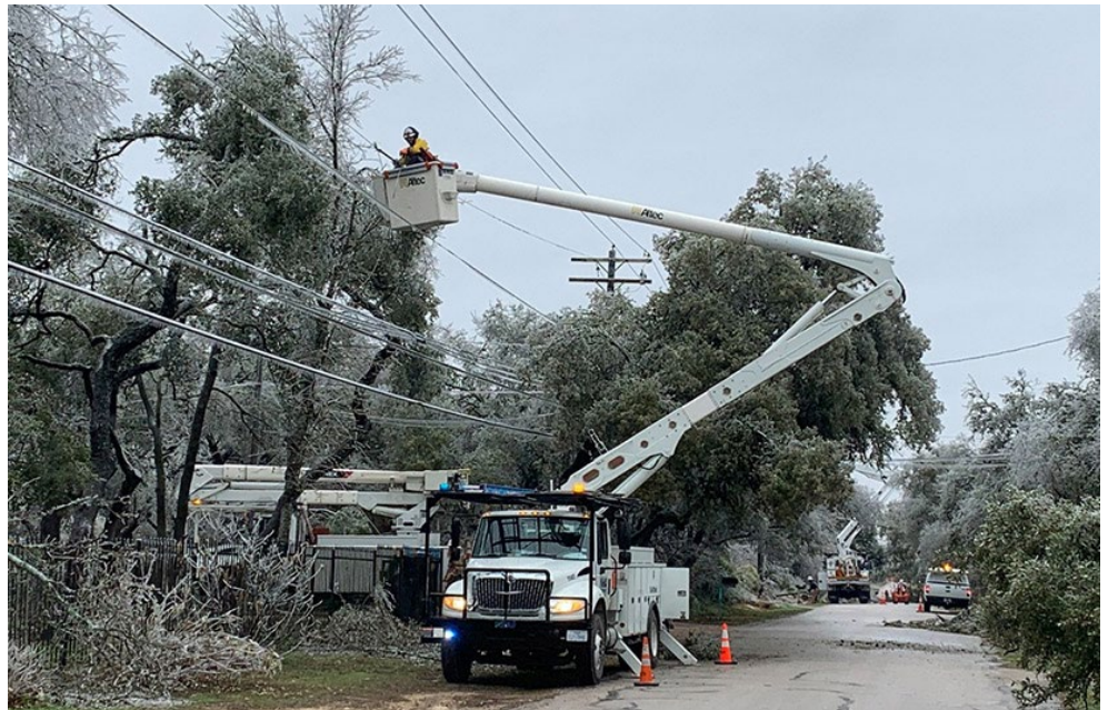
Austin Energy crews at work restoring service. | Austin Energy
