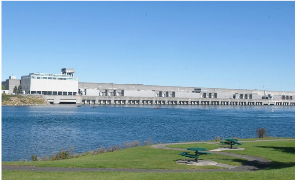
The New York Power Authority's St. Lawrence Power Project is shown in Massena, N.Y. Gov. Kathy Hochul is proposing an expansion of NYPA's role in the state's clean energy transition. | The New York Power Authority
