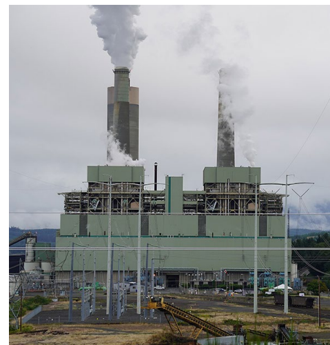
Washington’s new cap-and-trade rules apply to nearly all GHG emitters in the state, including TransAlta’s coal-fired Centralia Power Plant. | Steven Baltakatei CC-BY-SA 4.0, via Wikimedia Commons
