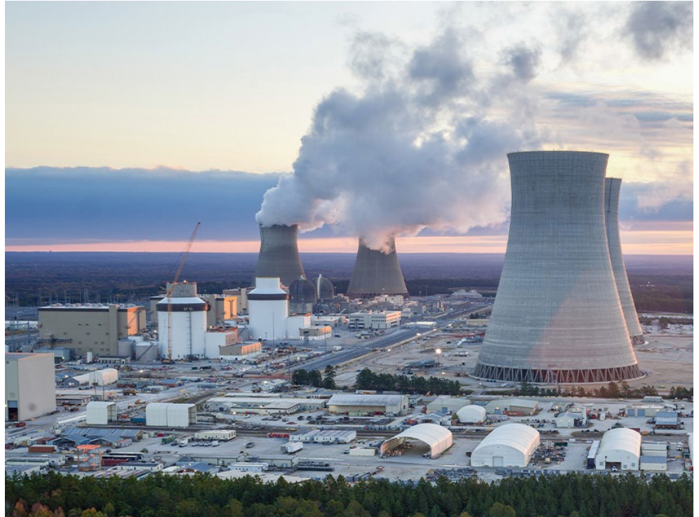
The Vogtle nuclear plant near Waynesboro, Ga. The original units, Vogtle 1 and 2, are in the background. The new units, 3 and 4, are in the foreground. | Georgia Power Company
