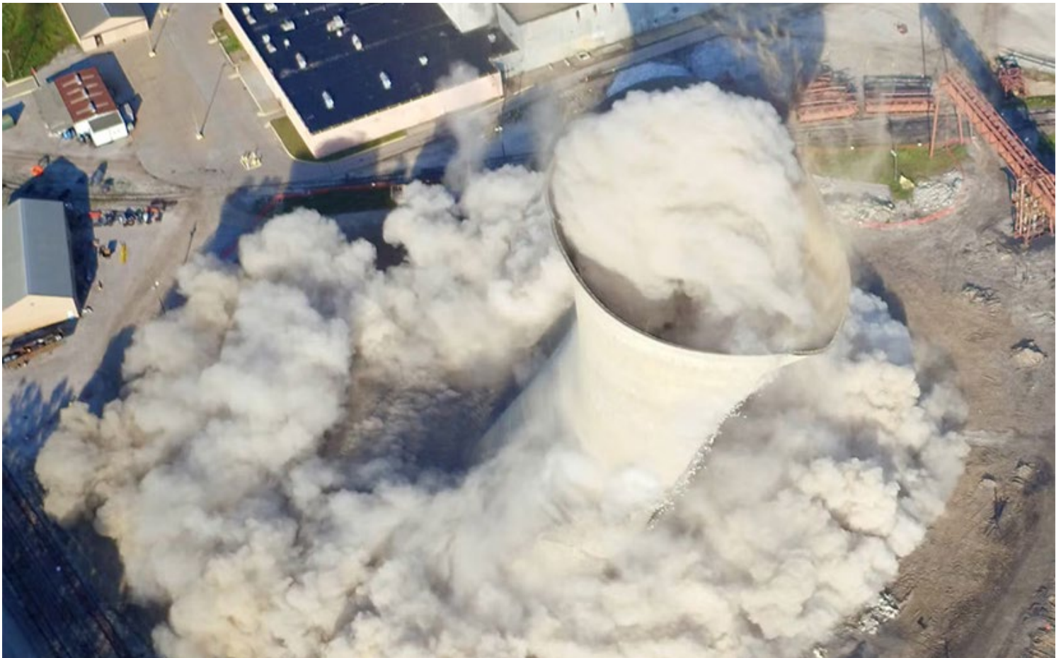
Implosion of a Big Sandy cooling tower in 2016 | Independence Demolition
