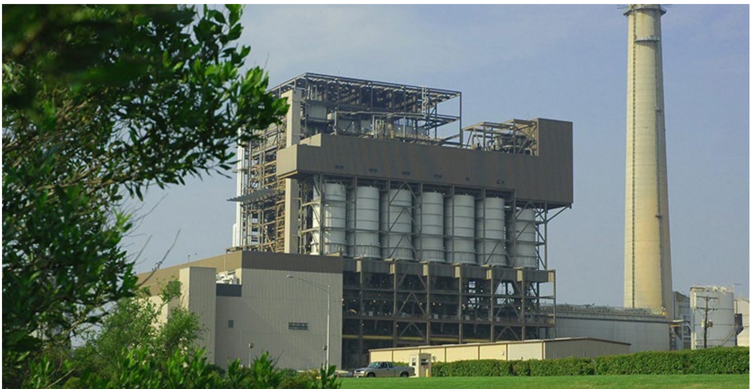
Pirkey Power Plant | Oklahoma Municipal Power Authority
