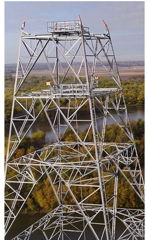
Ameren's Illinois Rivers project under construction | Ameren
