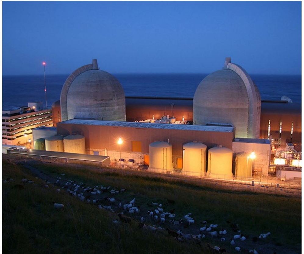
Diablo Canyon Power Plant sits on the coast of Central California. | PG&E
