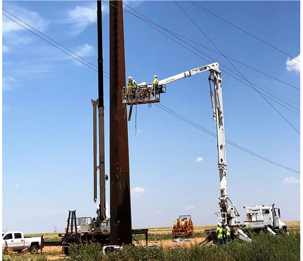
Line crew works on an Xcel Energy transmission line. | Xcel Energy
