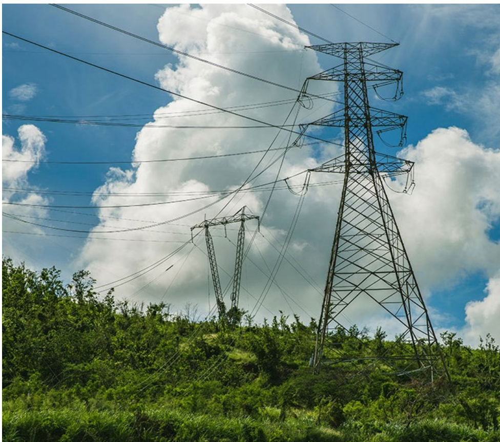
Damaged transmission lines in Puerto Rico after Hurricane Maria | Shutterstock
