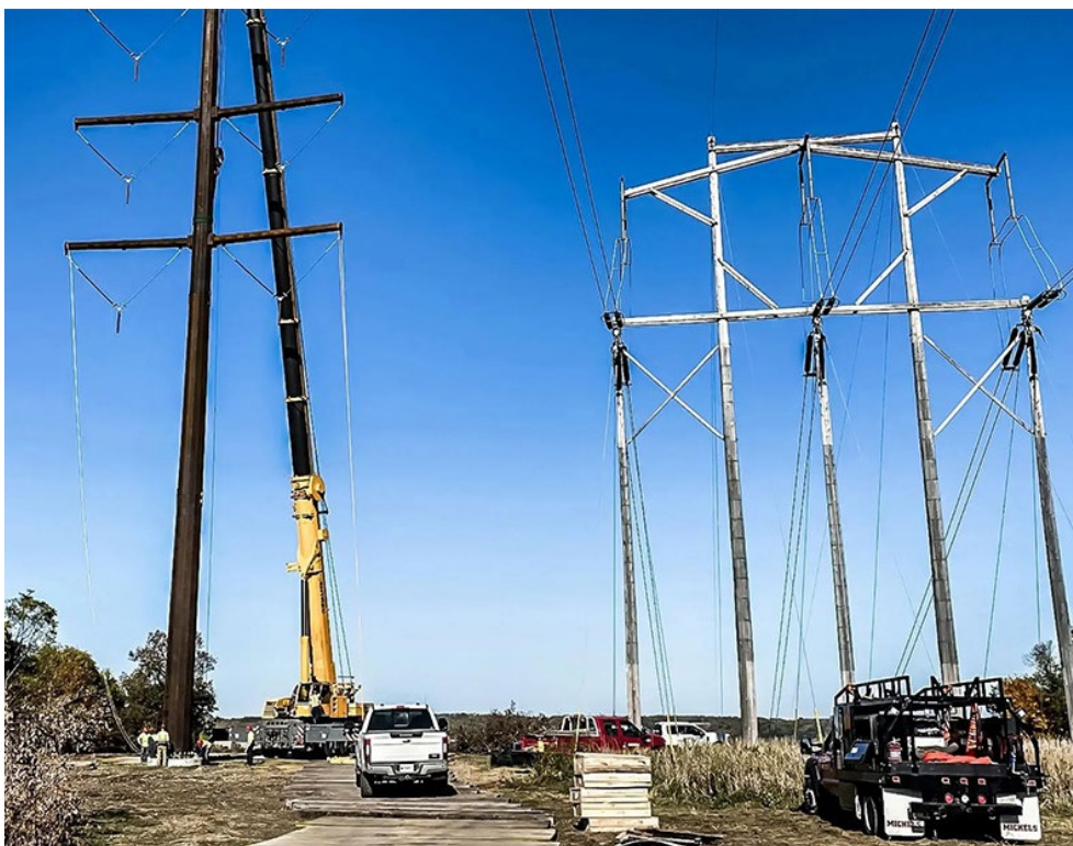
Construction of the Huntley-Wilmarth transmission line project in Minnesota | Michels Corporation
