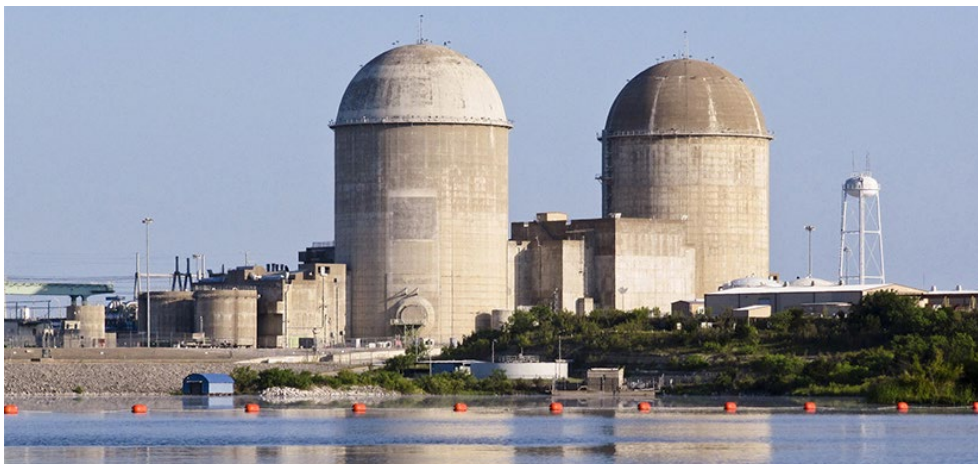
Luminant's Comanche Peak Nuclear Power Plant | Vistra
