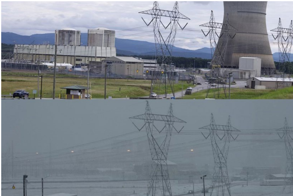
Entergy Arkansas' Arkansas Nuclear One plant pictured within the span of a few days in January 2023 | Entergy Arkansas
