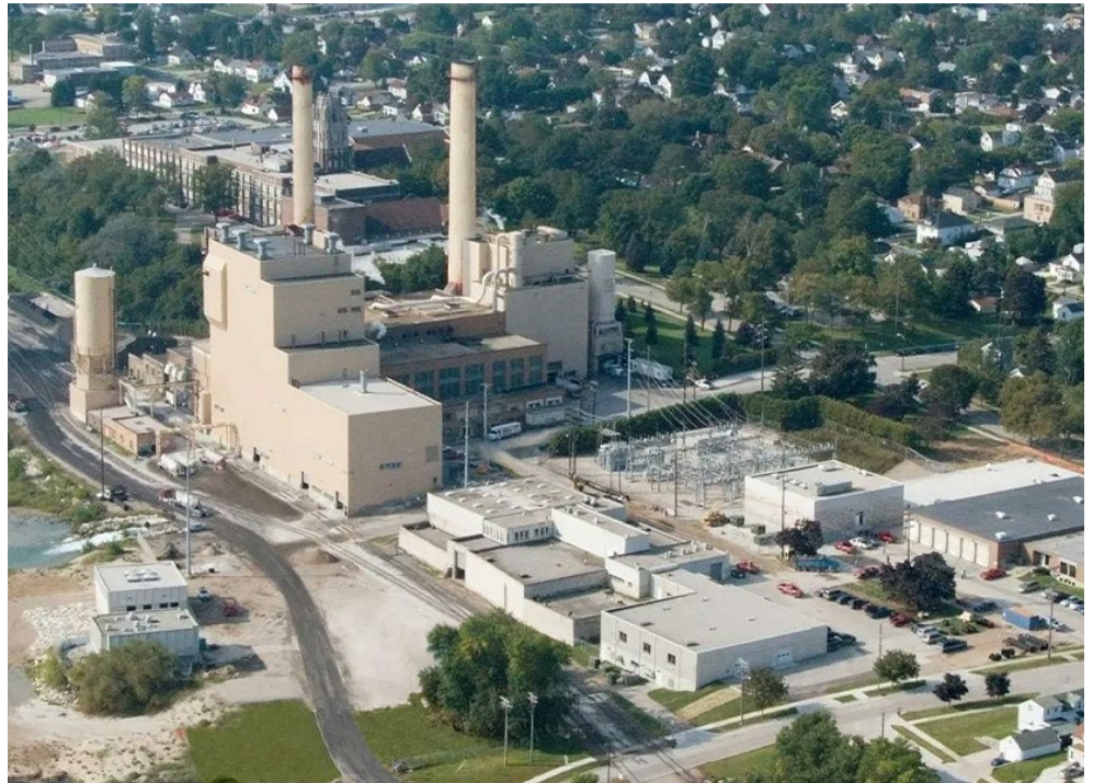
Manitowoc Public Utilities' Lakefront power plant | Manitowoc Public Utilities
