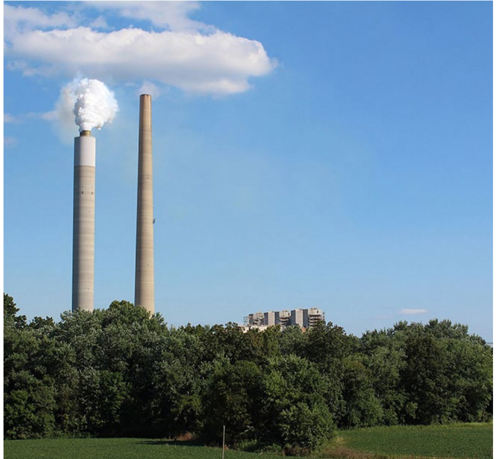
Ohio Valley Electric Corp.'s Kyger Creek Power Plant | FunksBrother, CC BY-SA 4.0, via Wikimedia Commons
