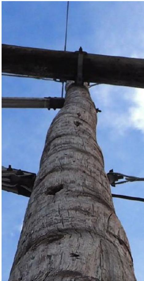
National Grid plans to spend an estimated \$138 million to replace 178 wood structures with new steel structures on its 115-kV transmission line between the Harriman #8 substation in Readsboro, Vt., and the Adams #21 substation in Adams, Mass., including this damaged wood utility pole. | *National Grid*
