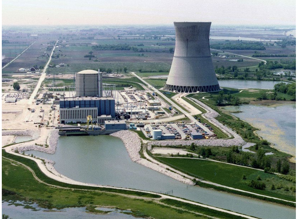
Davis-Besse nuclear plant in northern Ohio | NRC
