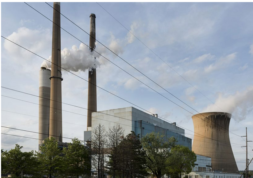
Pleasants Power Station in Belmont, W.Va. | Library of Congress
