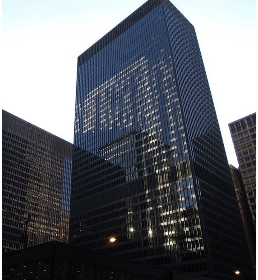
Federal Building and Dirksen United States Courthouse in downtown Chicago | Ken Lund, CC BY-SA 2.0, via Wikimedia Commons
