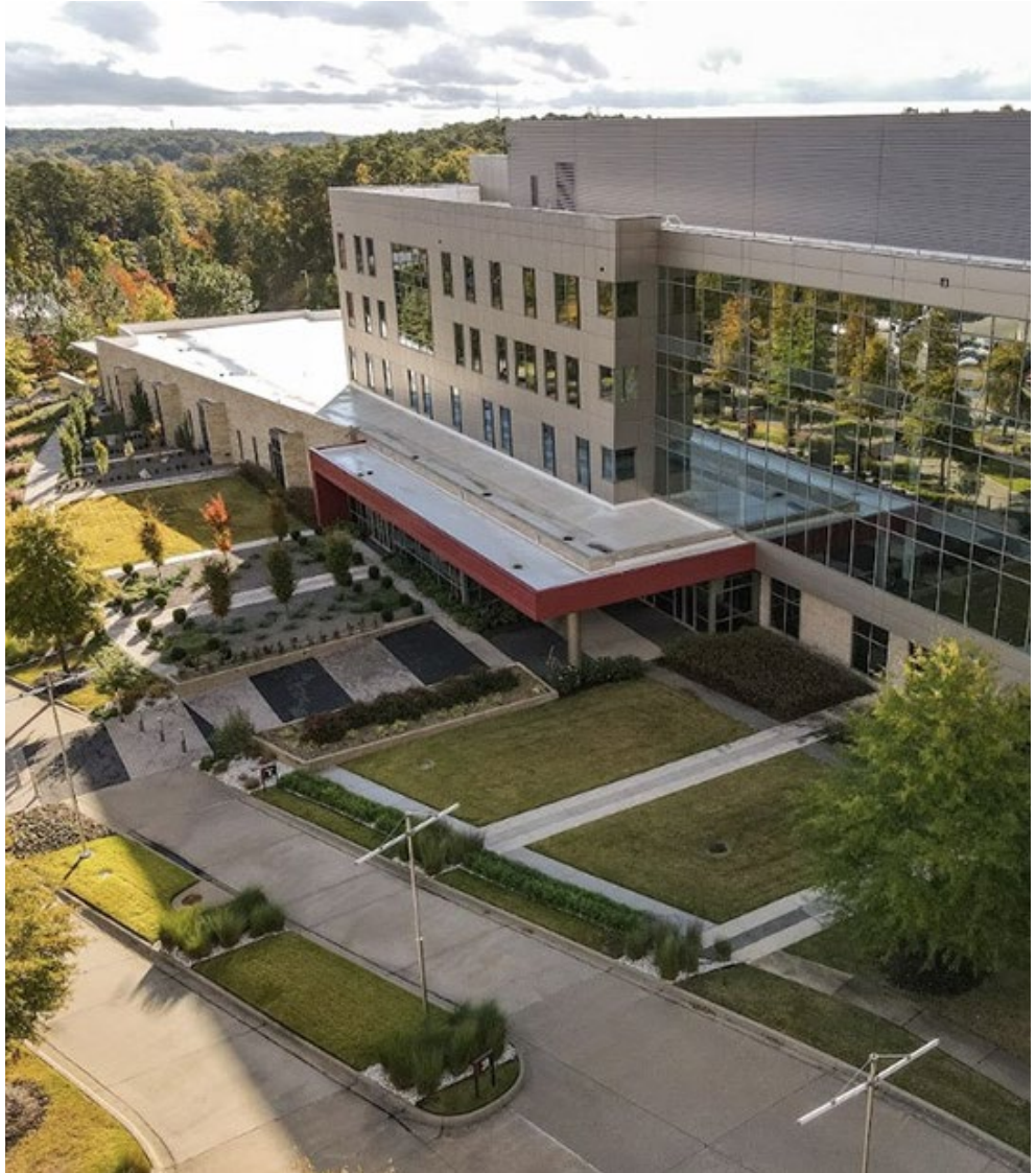
SPP headquarters in Little Rock, Ark. | SPP
