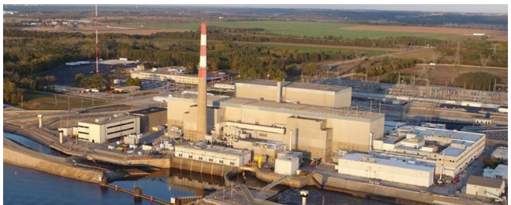
Quad Cities Generating Station, Illinois | Constellation Energy
