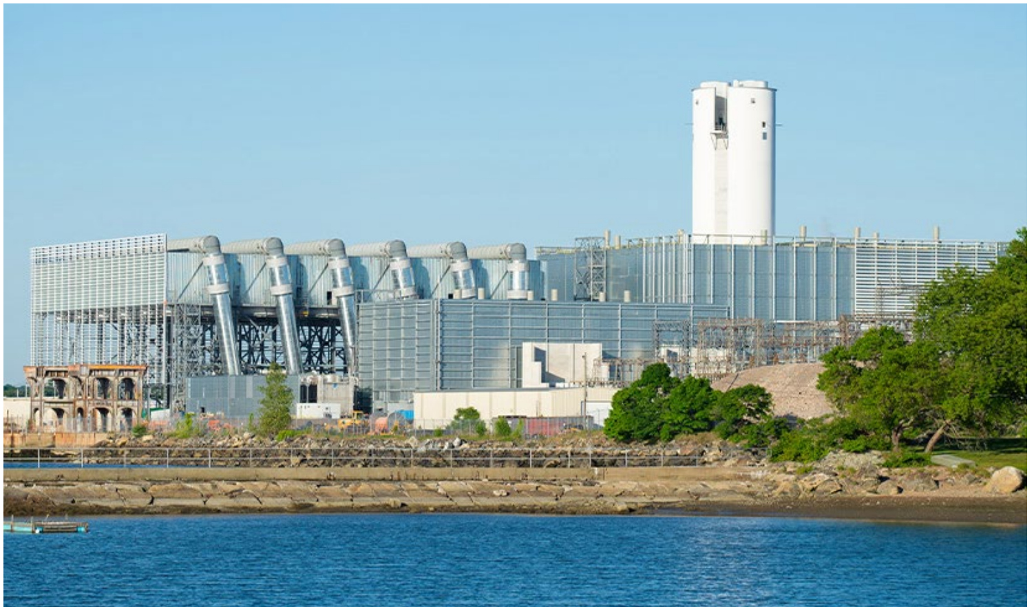
Salem Harbor Power Station, a gas-fired generating plant in Salem, Mass. | Fletcher, CC BY-SA 4.0, via Wikimedia Commons
