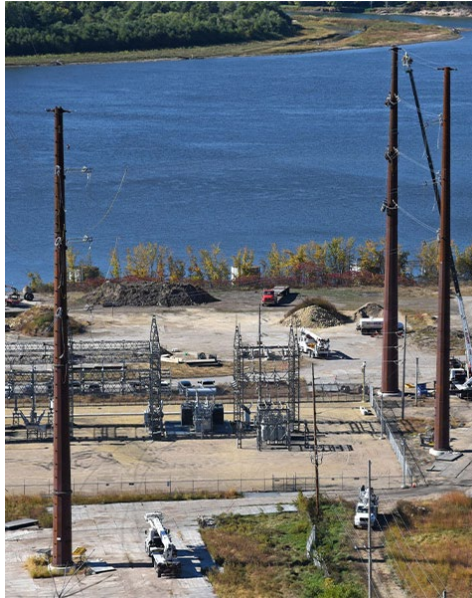
The Cardinal-Hickory Creek line under construction | ATC and ITC Midwest
