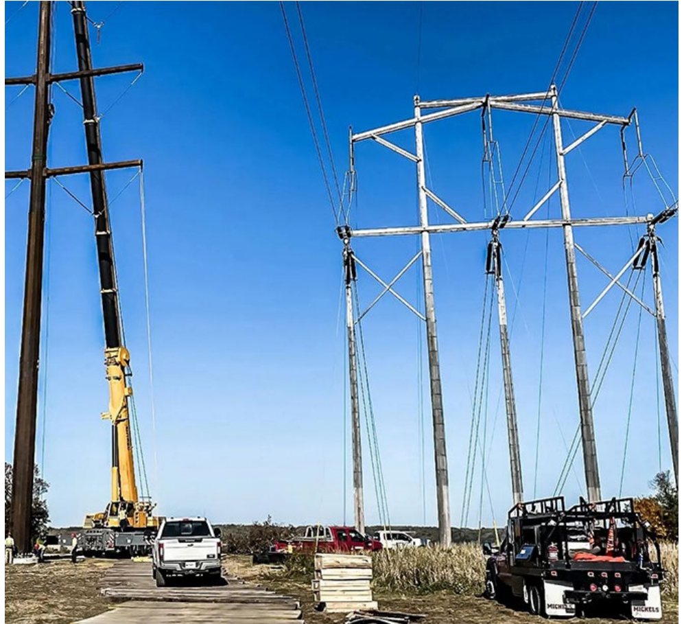
Construction of the Huntley-Wilmarth transmission line project in Minnesota | Michels Corporation
