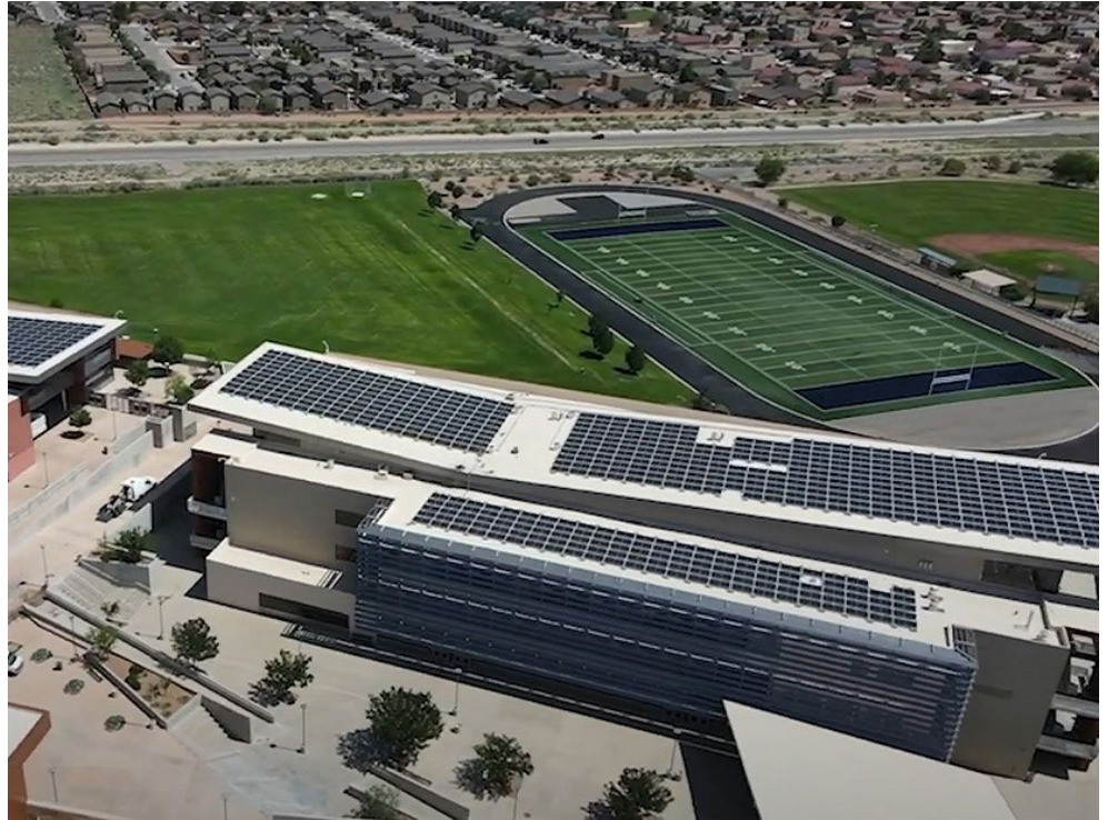
The 850-kW solar system, with storage, has been complete but unable to interconnect to the local distribution system since August of 2022 because of a range of interconnection bottlenecks and supply chain and workforce delays. | Albuquerque Public Schools
