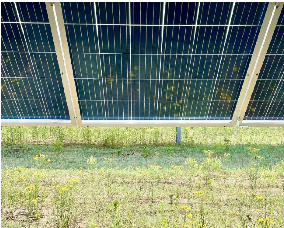
Pollinator habitat under a Minnesota Power solar facility | Minnesota Power
