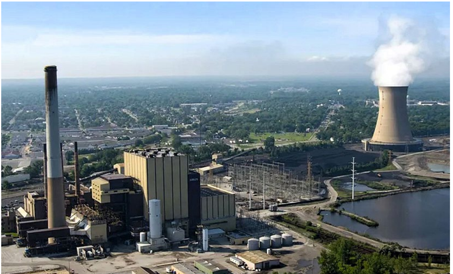
Northern Indiana Public Service Co.'s Michigan City generating station will shutter in the 2026-2028 time frame | NIPSCO
