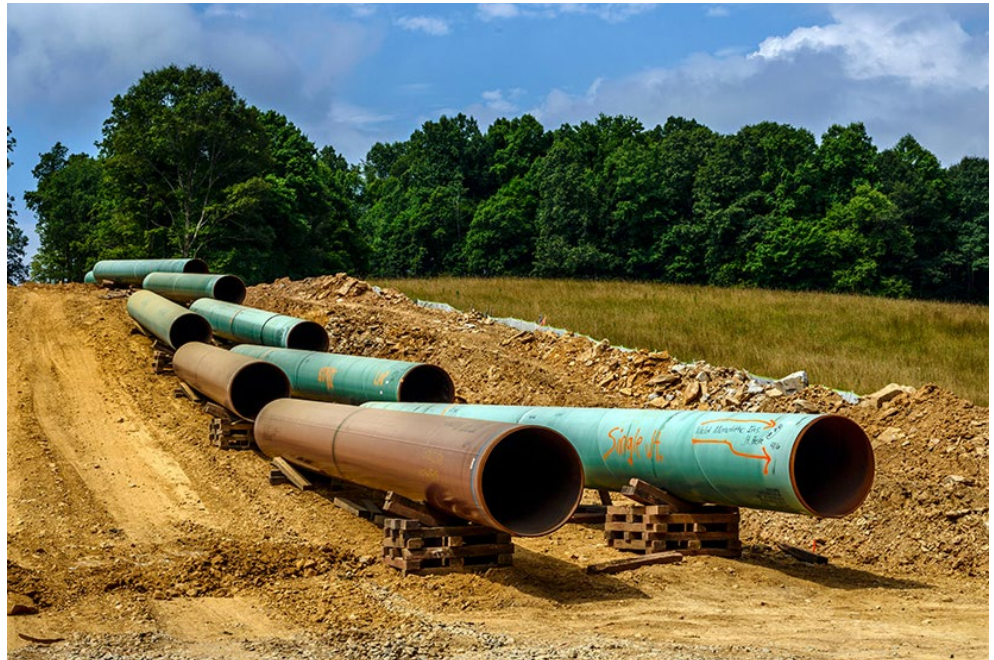
Construction of the Mountain Valley Pipeline | Shutterstock
