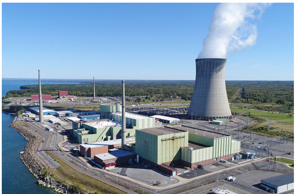
The Nine Mile Point nuclear station is shown in New York. | Constellation
