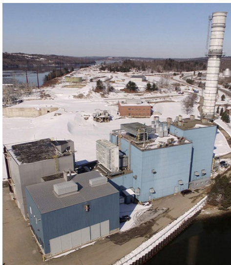
The Bucksport Power Station | JERA
