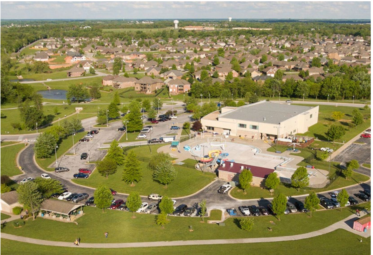
GridLiance High Plains owns about 10 miles of transmission lines and related facilities in Nixa, Mo. | City of Nixa, Mo.
