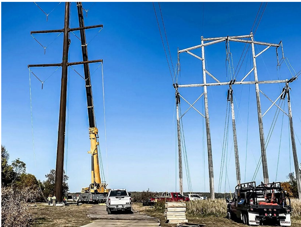
Construction of the Huntley-Wilmarth transmission line project in Minnesota | Michels Corporation
