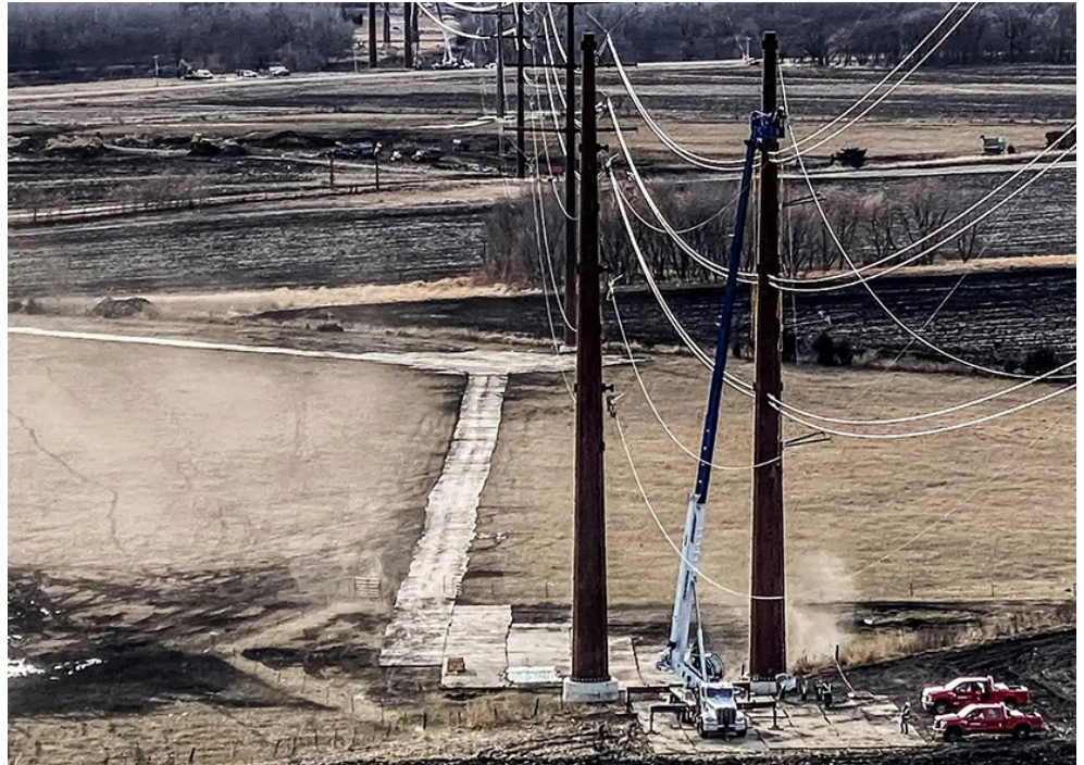
Construction of the Huntley-Wilmarth transmission line project in Minnesota | Michels Corporation
