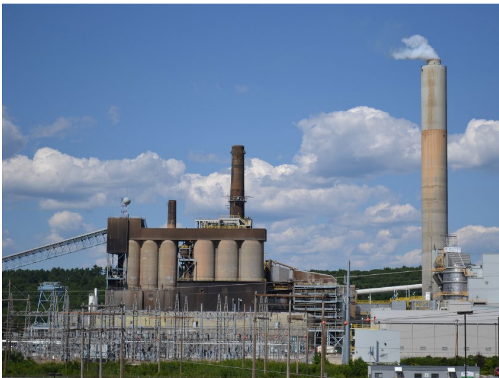
The Merrimack Station in New Hampshire, the last coal-fired power plant in New England | SayCheeeeeese, CC0 1.0 Public Domain, via Wikipedia
