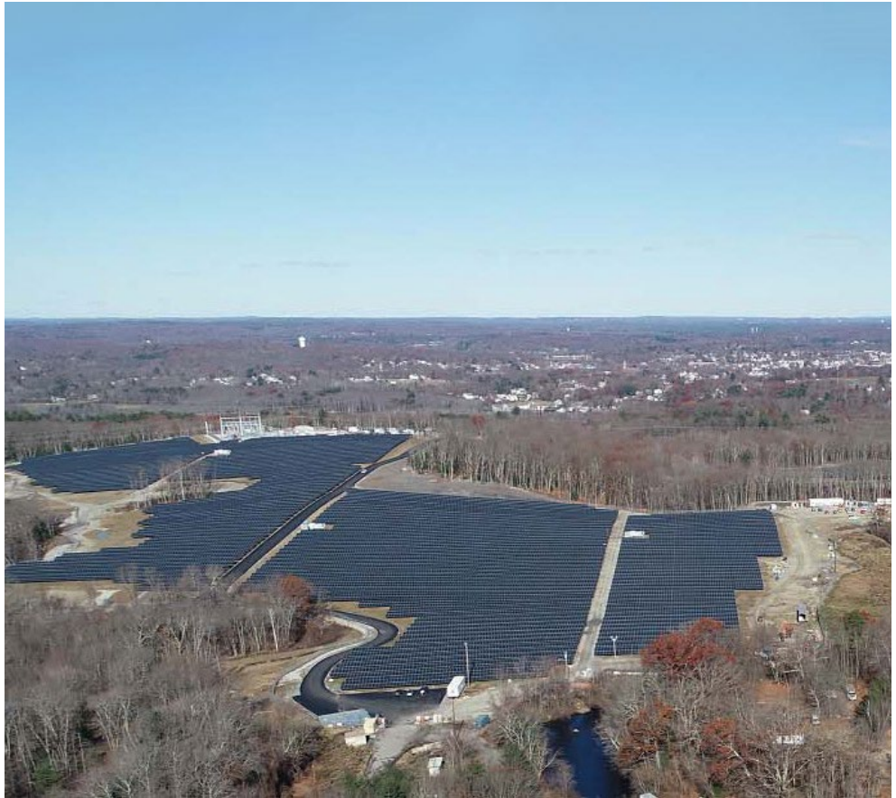
The Iron Mine solar project, owned and operated by Green Development | Green Development
