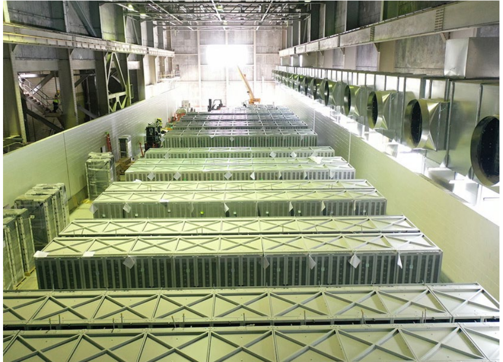
Moss Landing's turbine hall | LG Energy Solution
