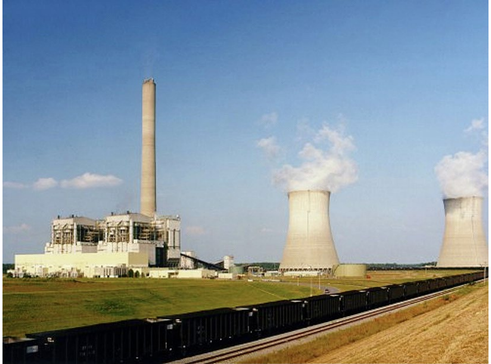
White Bluff power plant | Entergy Arkansas
