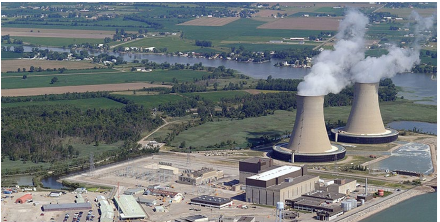
Fermi 2 nuclear plant | DTE Energy
