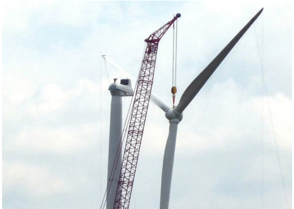
Construction of EDP Renewables' Harvest Ridge wind farm in Illinois | The Boldt Co.
