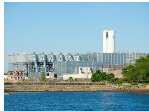
Salem Harbor Power Station, a gas-fired generating plant in Salem, Mass. | Fletcher, CC-BY-SA-4.0, via Wikipedia
