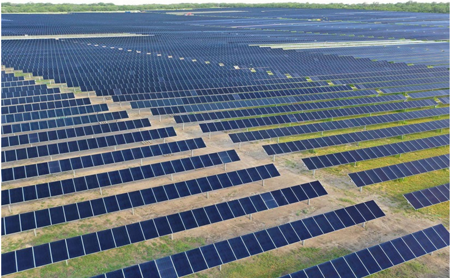
Solar energy is expected to produce about 12 GW during peak periods this fall. | Vistra Corp.
