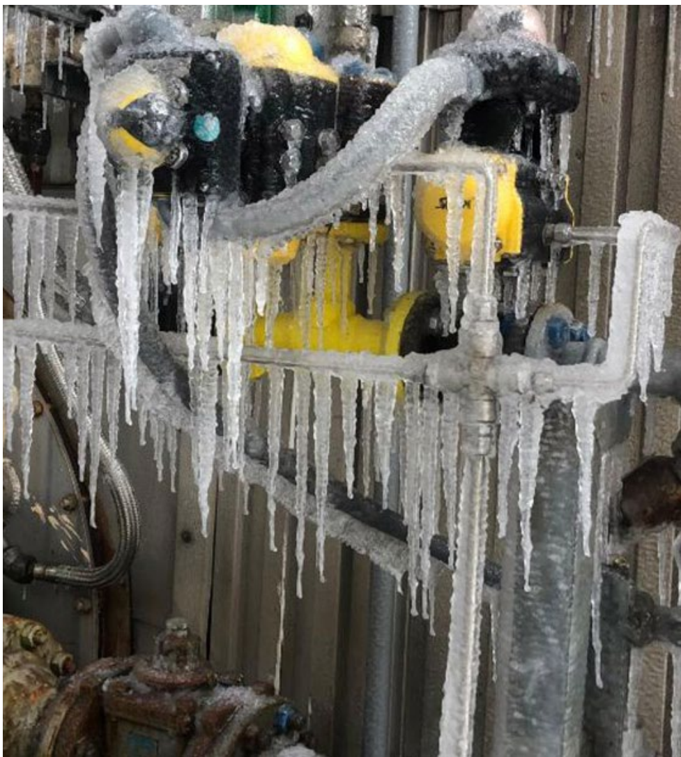
New weatherization rules are intended to prevent freezing issues like those during the 2021 winter storm. | Entergy
