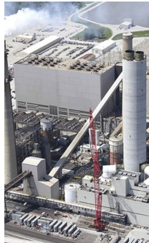
R.M. Schahfer Generating Station | NIPSCO
