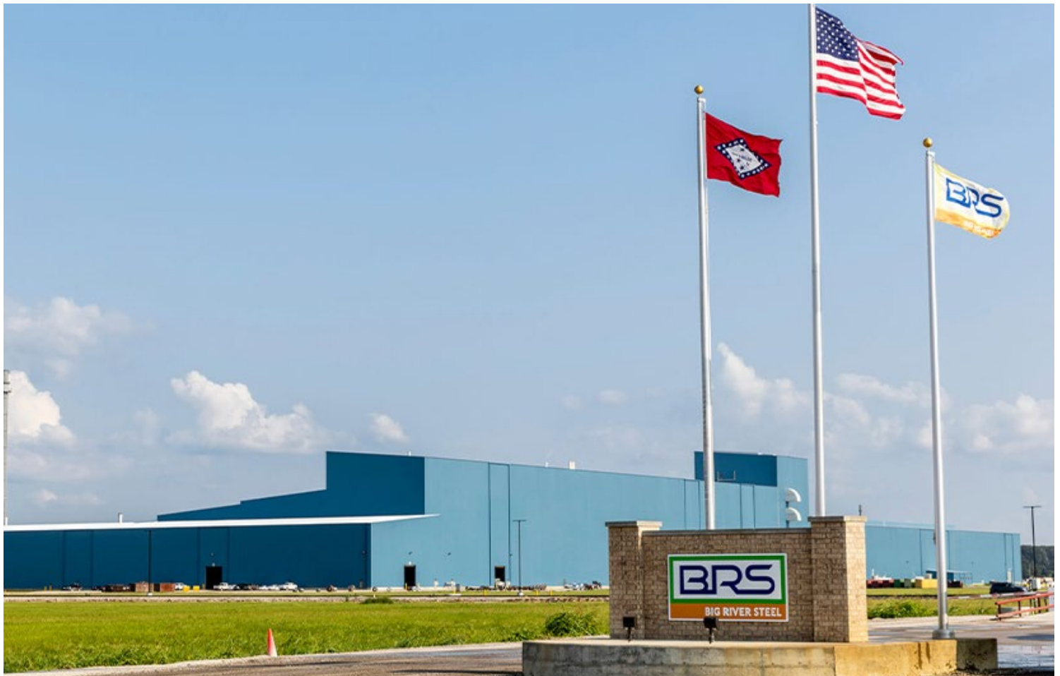
Big River Steel in Arkansas | Big River Steel
