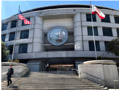
CPUC headquarters in San Francisco | © RTO Insider LLC
