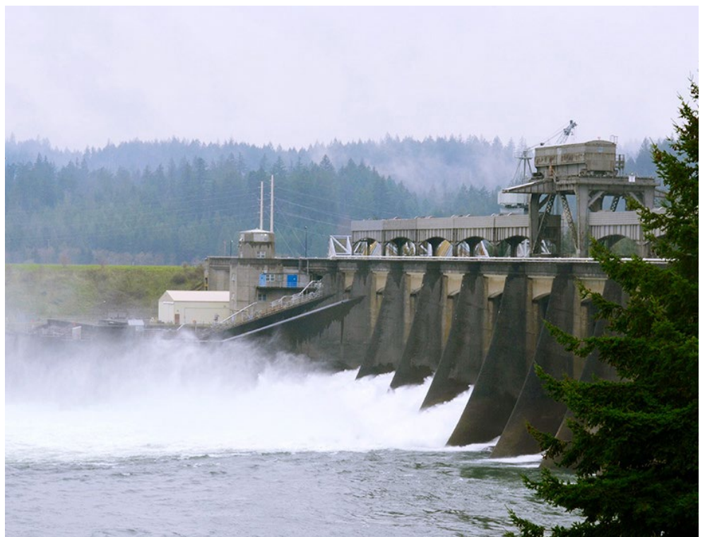
Spillway at BPA's Bonneville Dam. | © RTO Insider LLC
