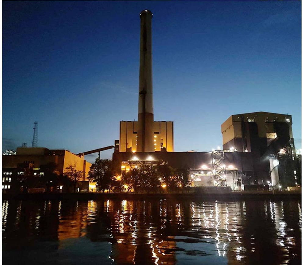
NIPSCO plans to shutter its Michigan City Generating Station in the 2026-2028 timeframe | © RTO Insider LLC
