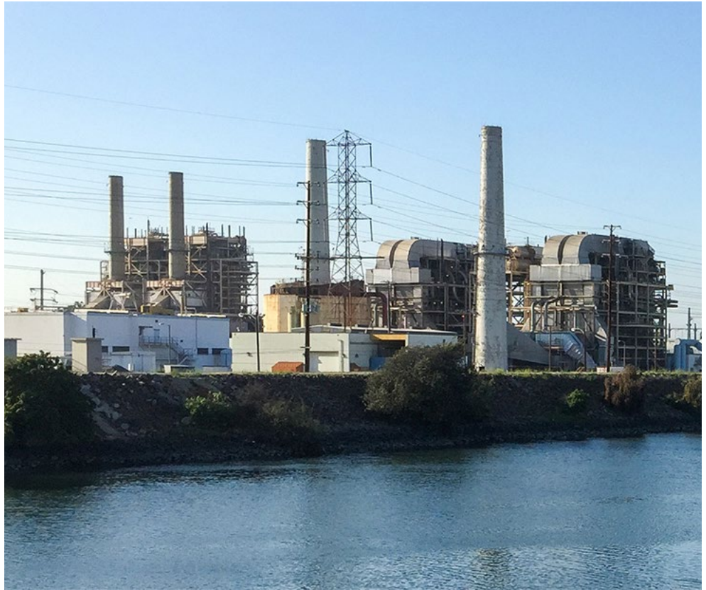
AES's Alamitos Energy Center in Long Beach, Calif. | The Greater Southwestern Exploration Company
