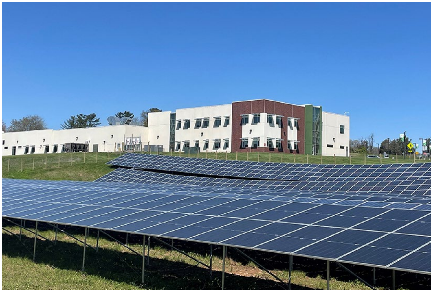
A solar array at the Workforce Training Center at Raritan Valley Community College in North Branch, N.J. | Raritan Valley Community College
