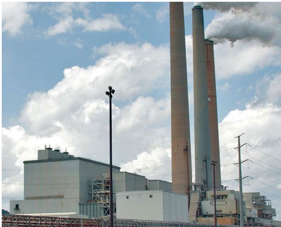
Mill Creek Generating Station | LG&E-KU
