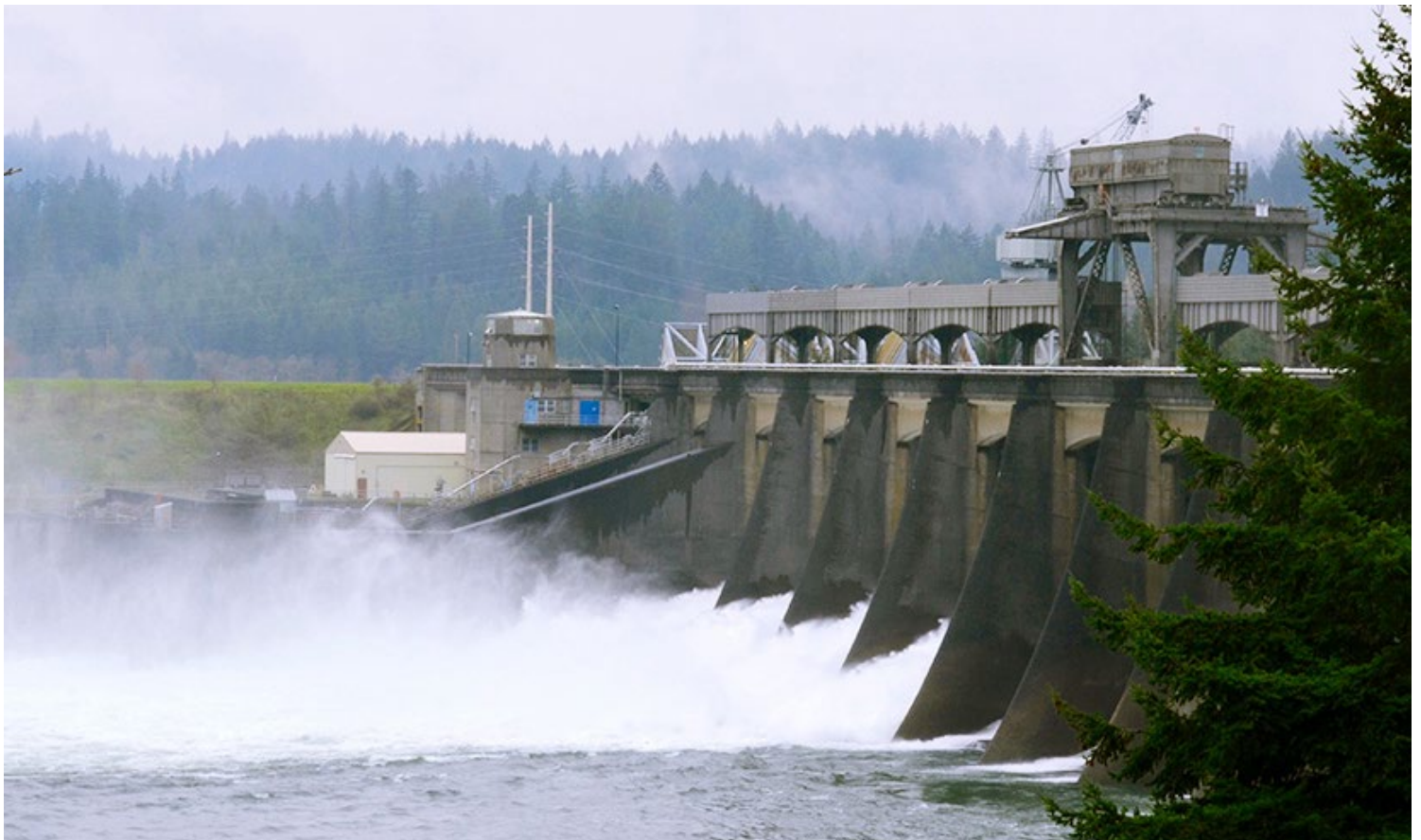
BPA's Bonneville Dam | © RTO Insider LLC
