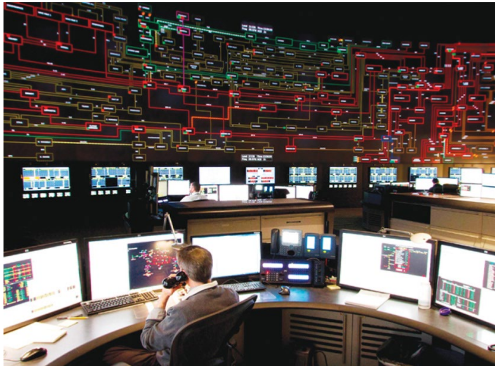
NYISO control room in Rensselaer, N.Y. | NYISO
