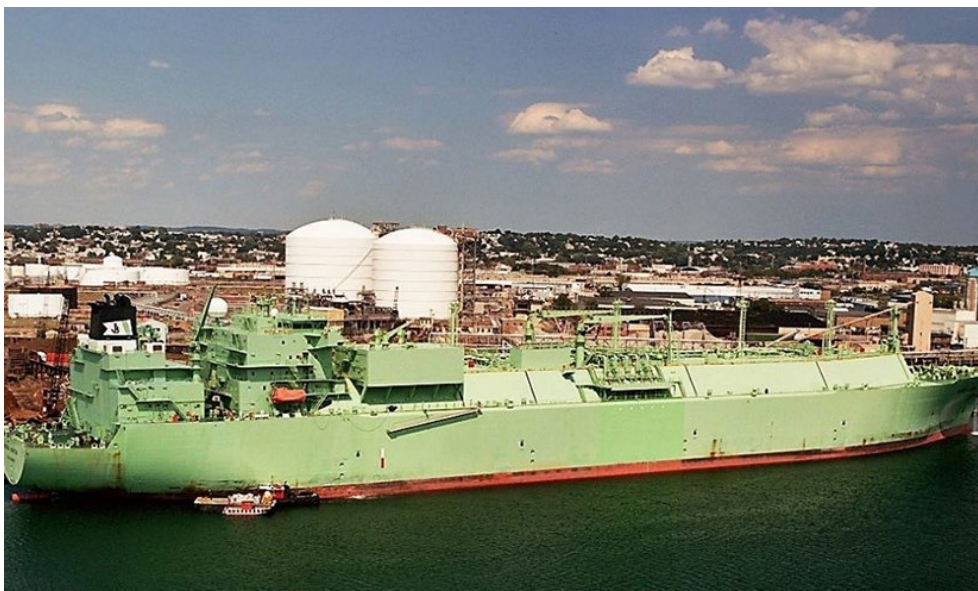
Everett LNG facility | Constellation Energy
