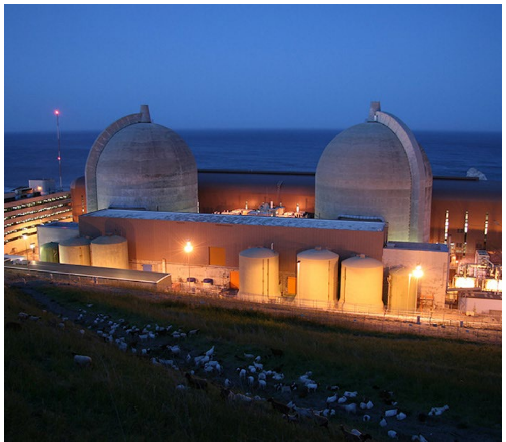
Diablo Canyon Power Plant sits on the coast of Central California. | PG&E
