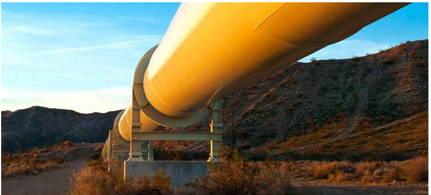
Calumet gas pipeline | Calumet
