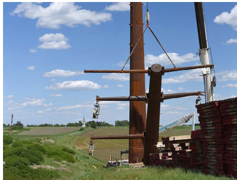
The Cardinal-Hickory Creek line under construction | ATC and ITC Midwest
