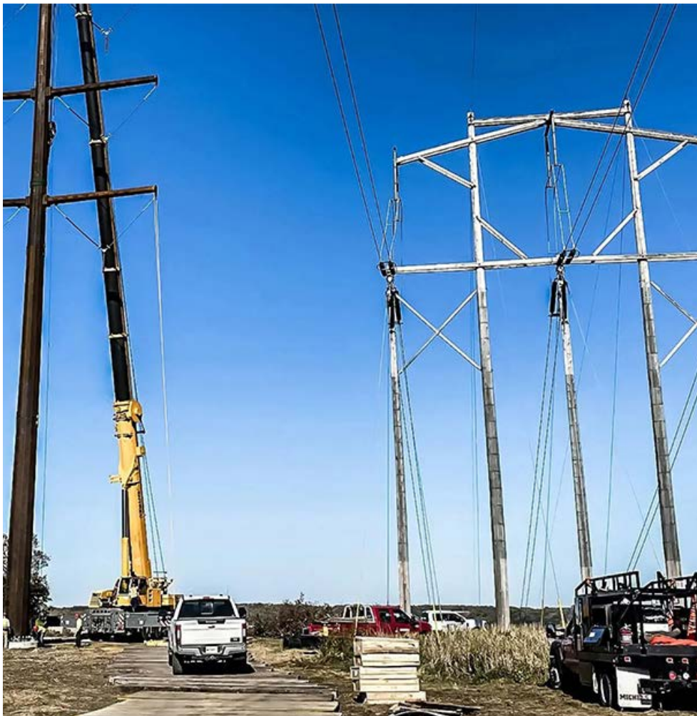
Construction of the Huntley-Wilmarth transmission line project in Minnesota | Michels Corporation
