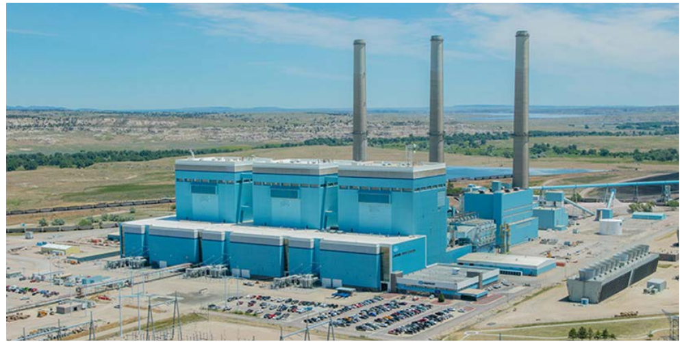
Laramie River Station, co-owned by Lincoln Electric System and three other utilities. | Basin Electric Power Cooperative
