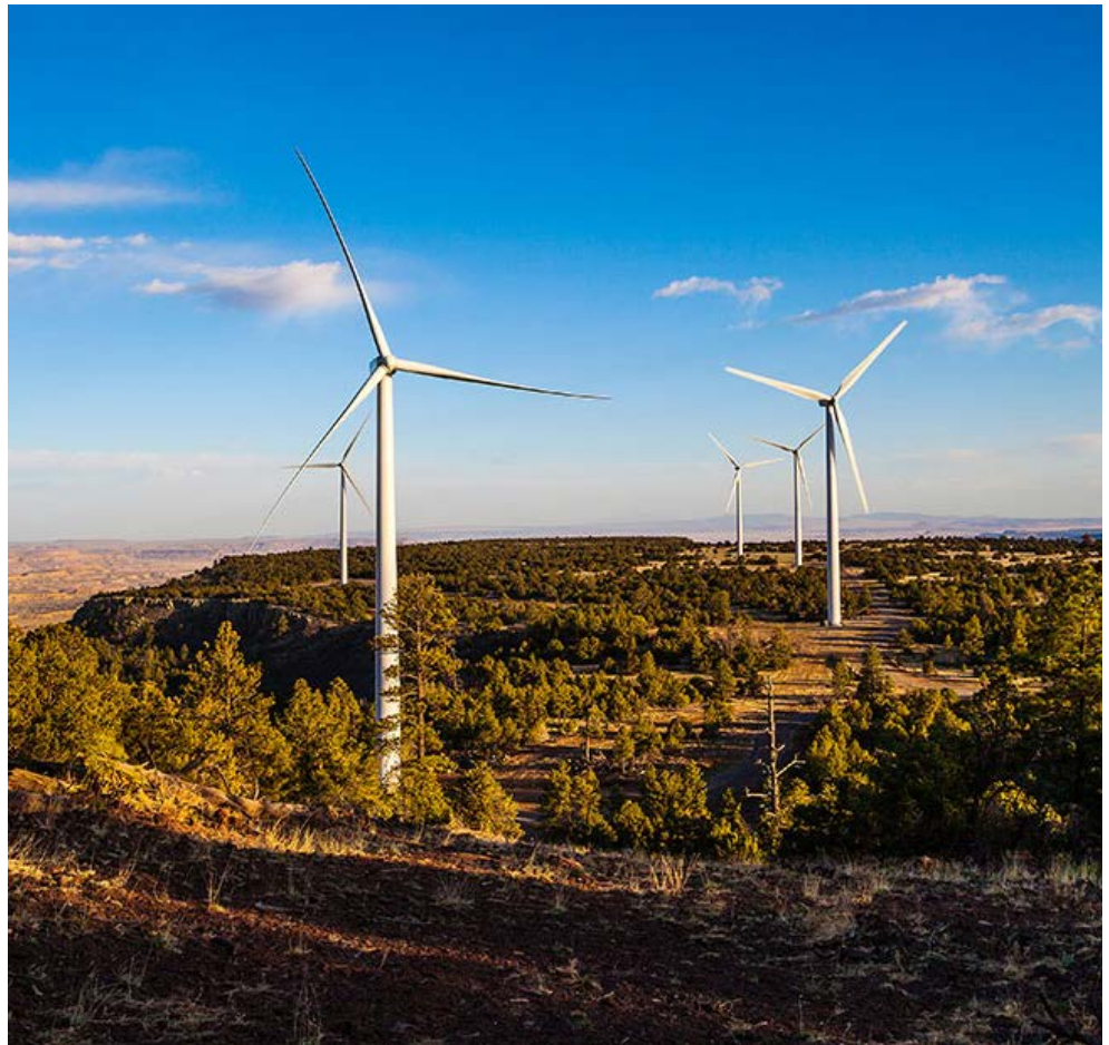
PNM wind turbines in New Mexico. Avangrid has called off its proposed acquisition of PNM Resources, the parent company of PNM, New Mexico's largest investor-owned utility. | Shutterstock
