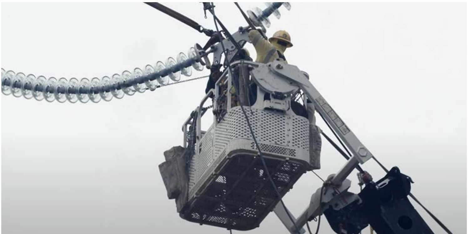
Work on ATC and Xcel's Badger Coulee Transmission project in 2018 | IBEW
