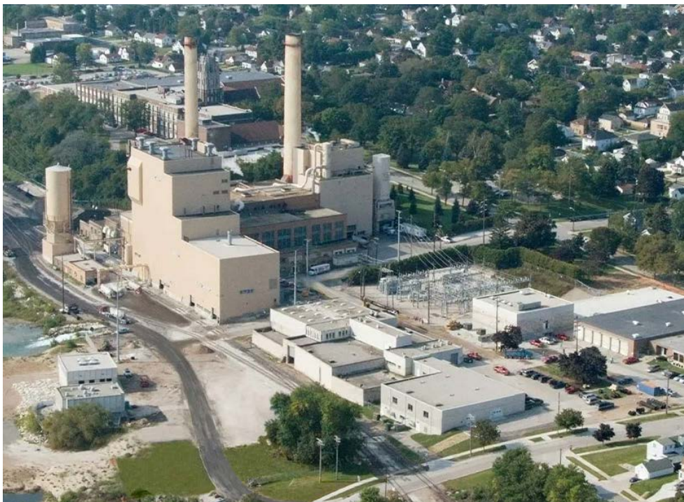
Manitowoc Public Utilities' Lakefront power plant | Manitowoc Public Utilities
