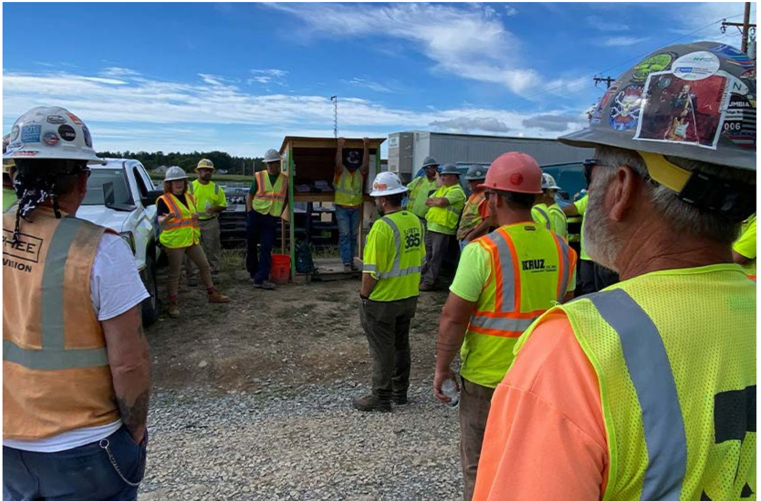
Workers prepare to begin construction on the Propel NY Energy project. | Propel NY Energy
