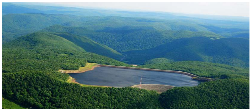
Brookfield Renewables' Bear Swamp hydro project | State of Massachusetts
