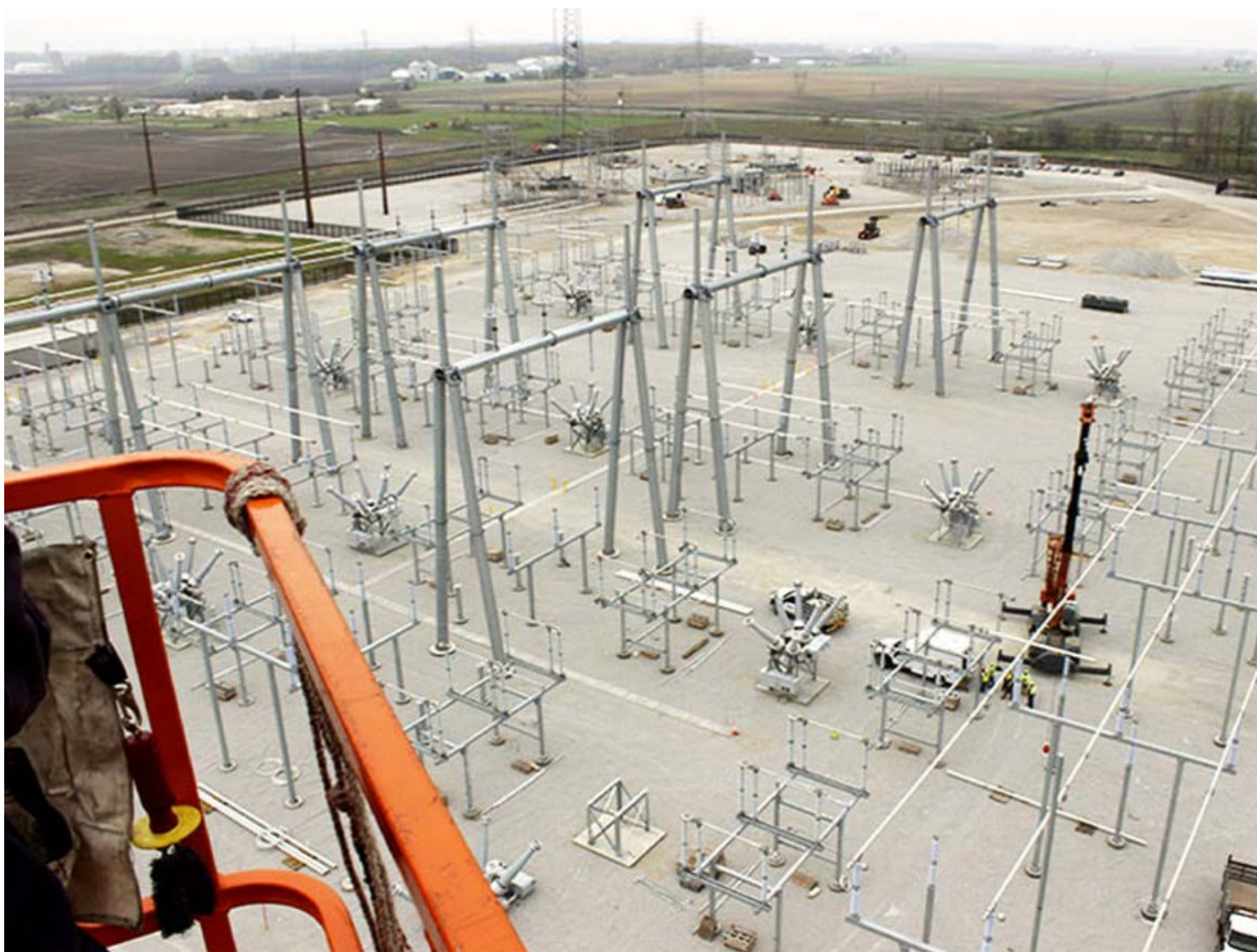
NIPSCO construction on the Reynolds substation in 2017 | NiSource
