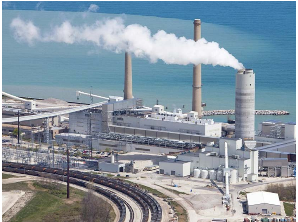
Oak Creek Power Plant | We Energies
