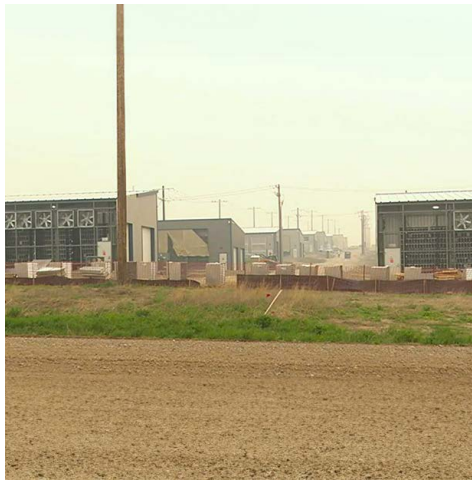
The Atlas Power Data Center in Williston | KFYR TV
