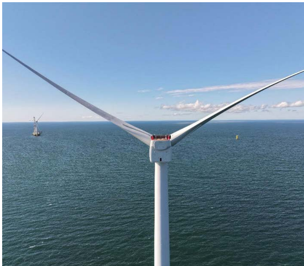
A turbine stands at the Vineyard Wind project south of Martha’s Vineyard, Massachusetts. | Worldview Films
