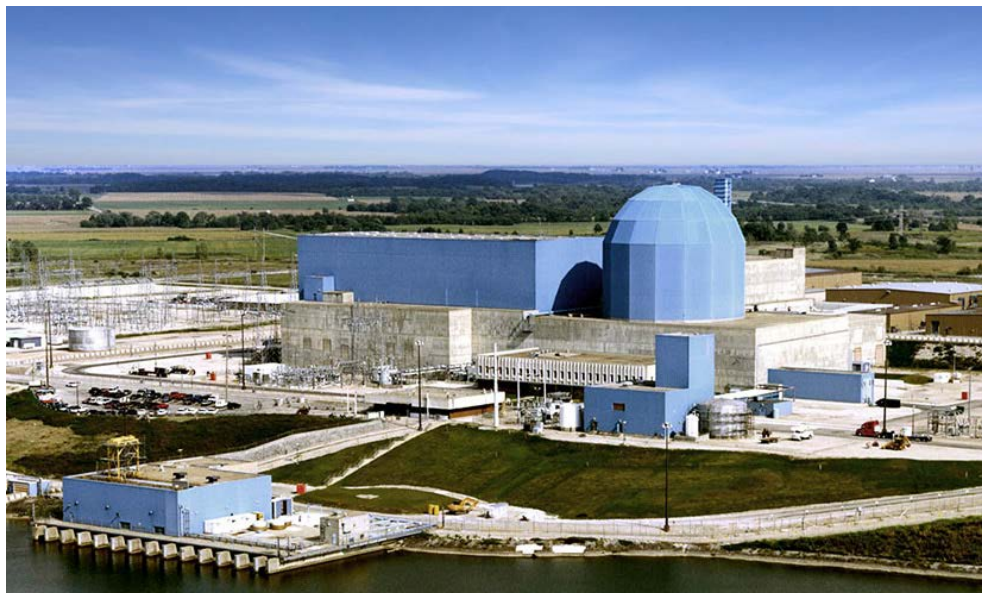
Constellation's nuclear power plant in Clinton, Ill., is shown. The company on Feb. 27 reported strong 2023 earnings and projected strong growth in large part due to its nuclear fleet. | Constellation Energy
