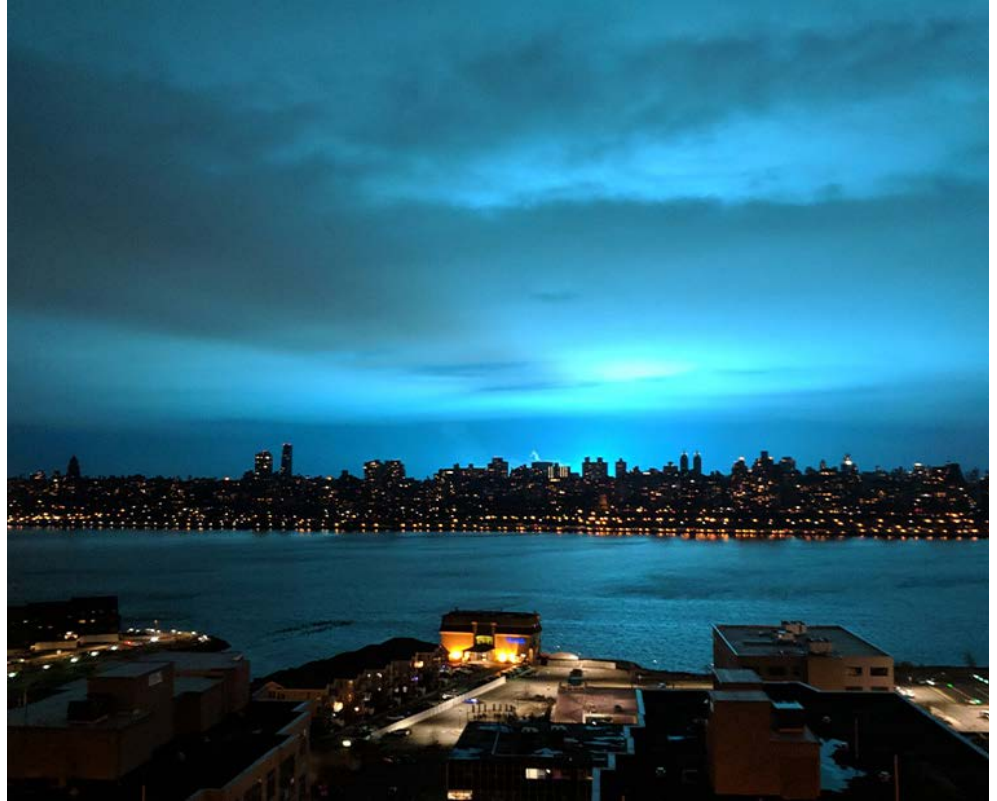
Con Edison transformer explosion in Queens from December 2018 | @prasad2011 via X
