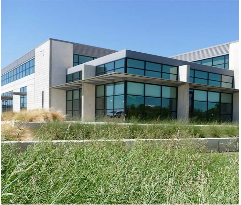
ERCOT headquarters in Austin, Texas | © RTO Insider LLC
