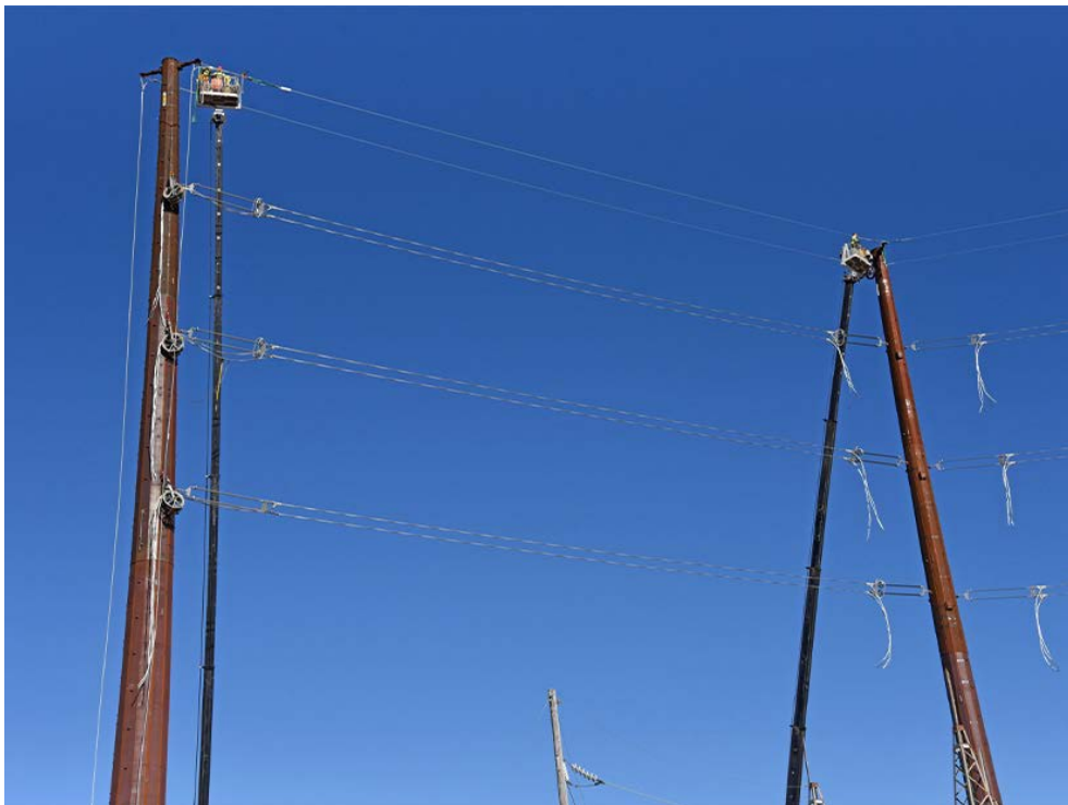
The Cardinal-Hickory Creek line under construction | ATC and ITC Midwest
