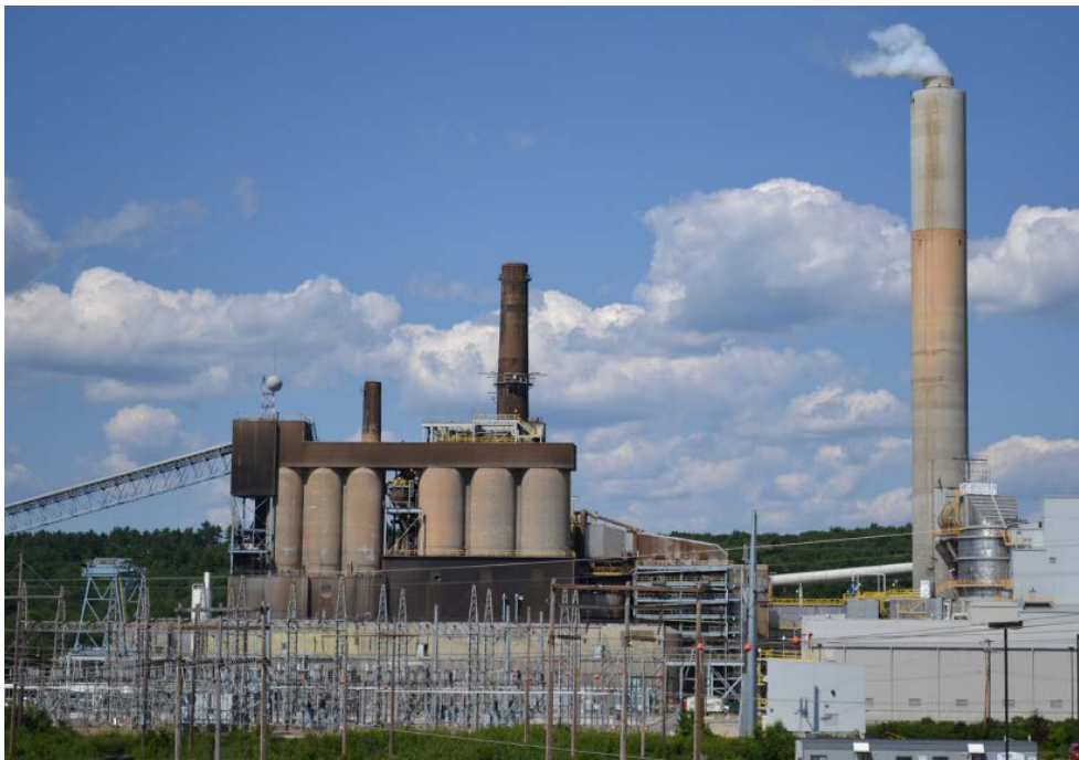
The Merrimack Station in New Hampshire, the last coal-fired power plant in New England | SayCheeeeeese , CC0 1.0 Public Domain, via Wikipedia
