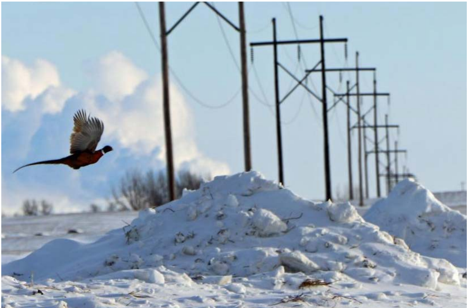
| Central Power Electric Cooperative
