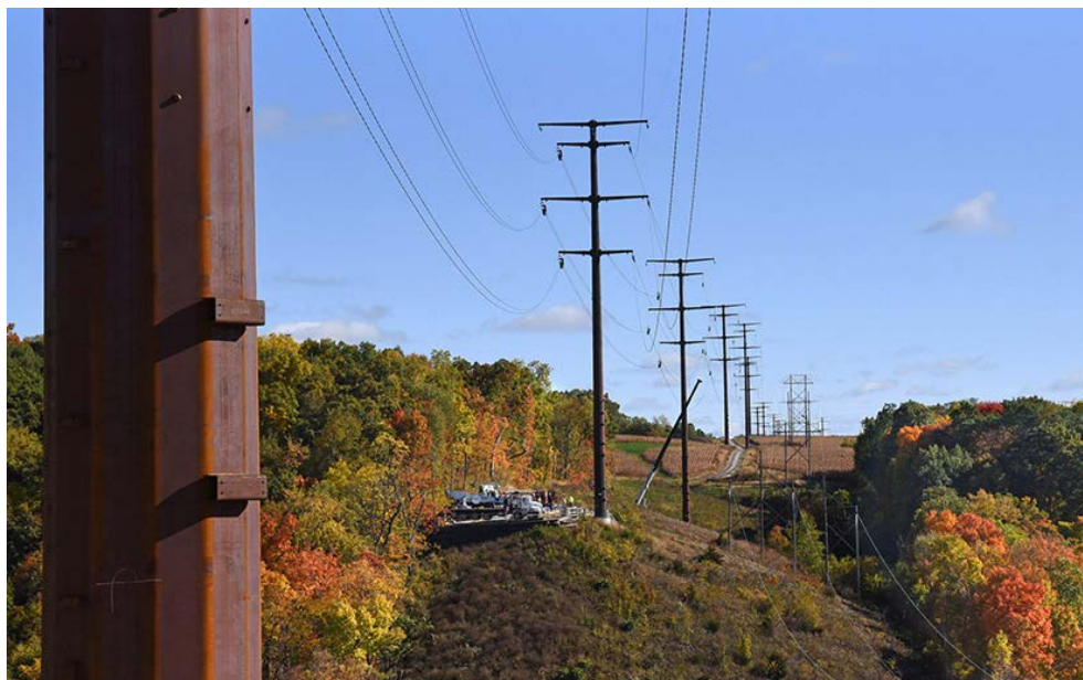
The Cardinal-Hickory Creek line under construction | ATC and ITC
