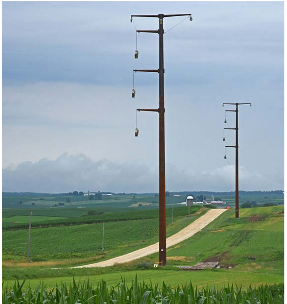
The Cardinal-Hickory Creek line under construction | ATC and ITC Midwest
