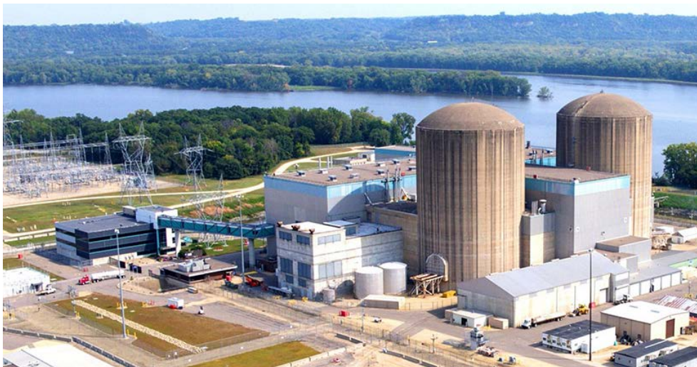
Prairie Island nuclear plant in Welch, Minn. | Xcel Energy
