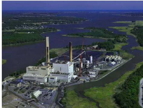
NRG's Indian River Generating Station in Delaware | NRG
