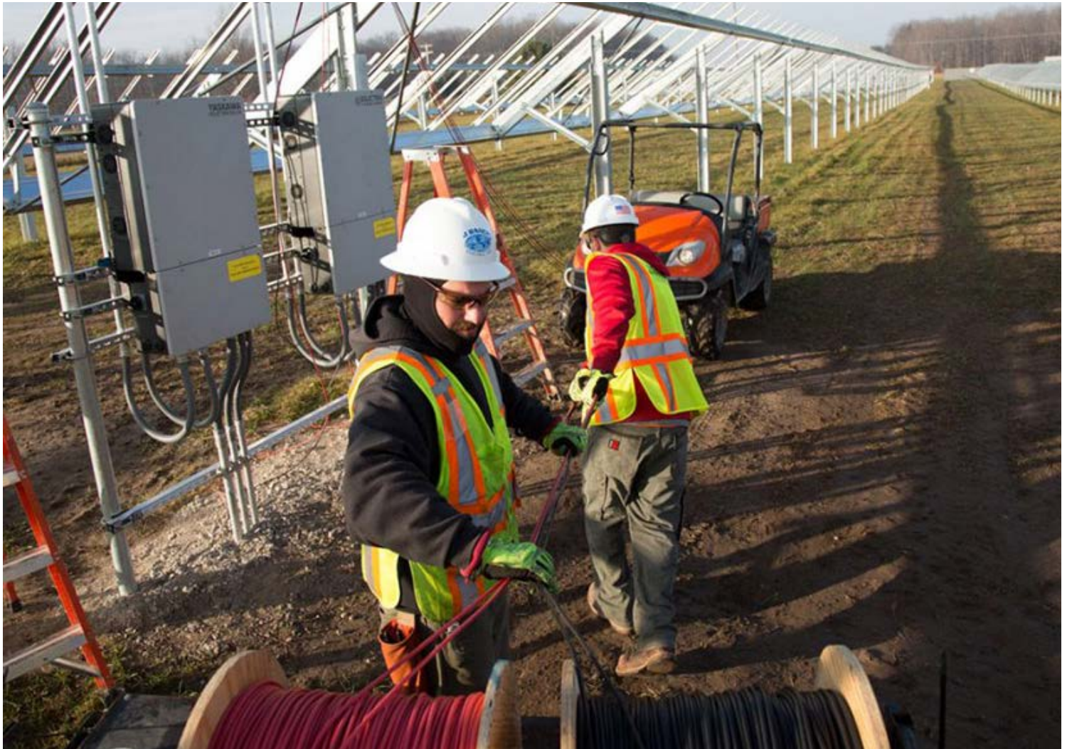
Solar array installation in Michigan for Wolverine Power Cooperative | J.Ranck Electric
