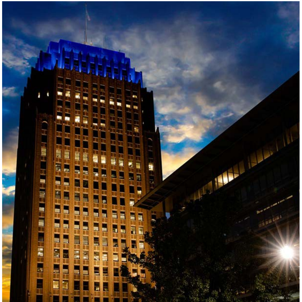
PPL headquarters in Allentown, Pa. | PPL
