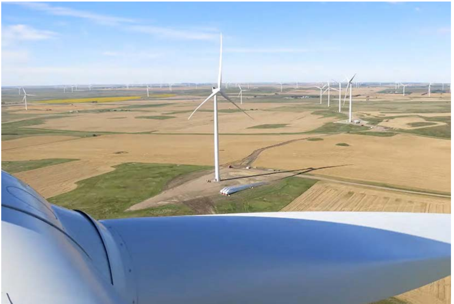
Minnesota Power's Bison Wind Energy Center in North Dakota | Allete
