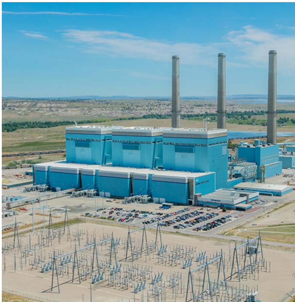
SPP is concerned EPA's final GHG rule will hasten the retirement of thermal resources. | Basin Electric
