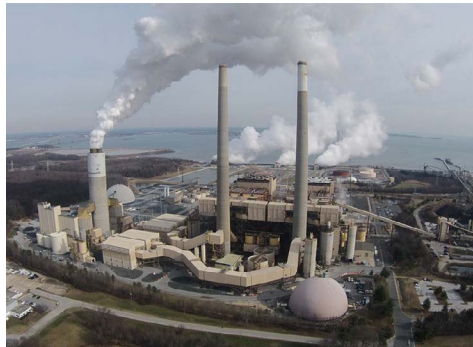
The Brandon Shores coal-fired power plant | Talen Energy
