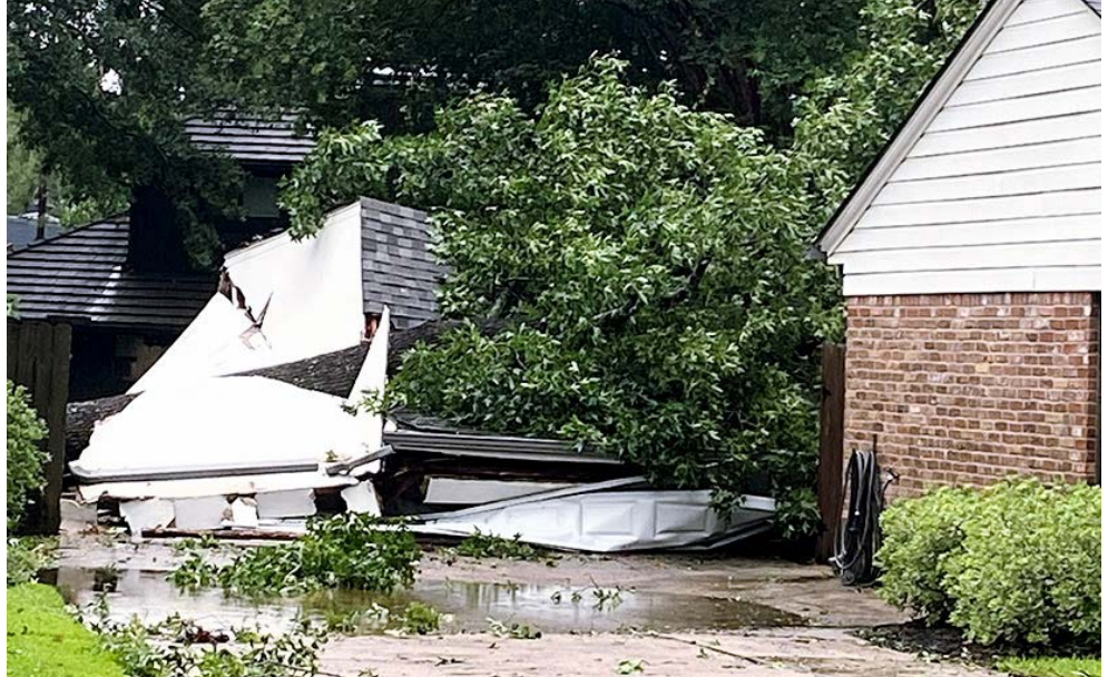
Garage crushed by downed tree. | © RTO Insider LLC
