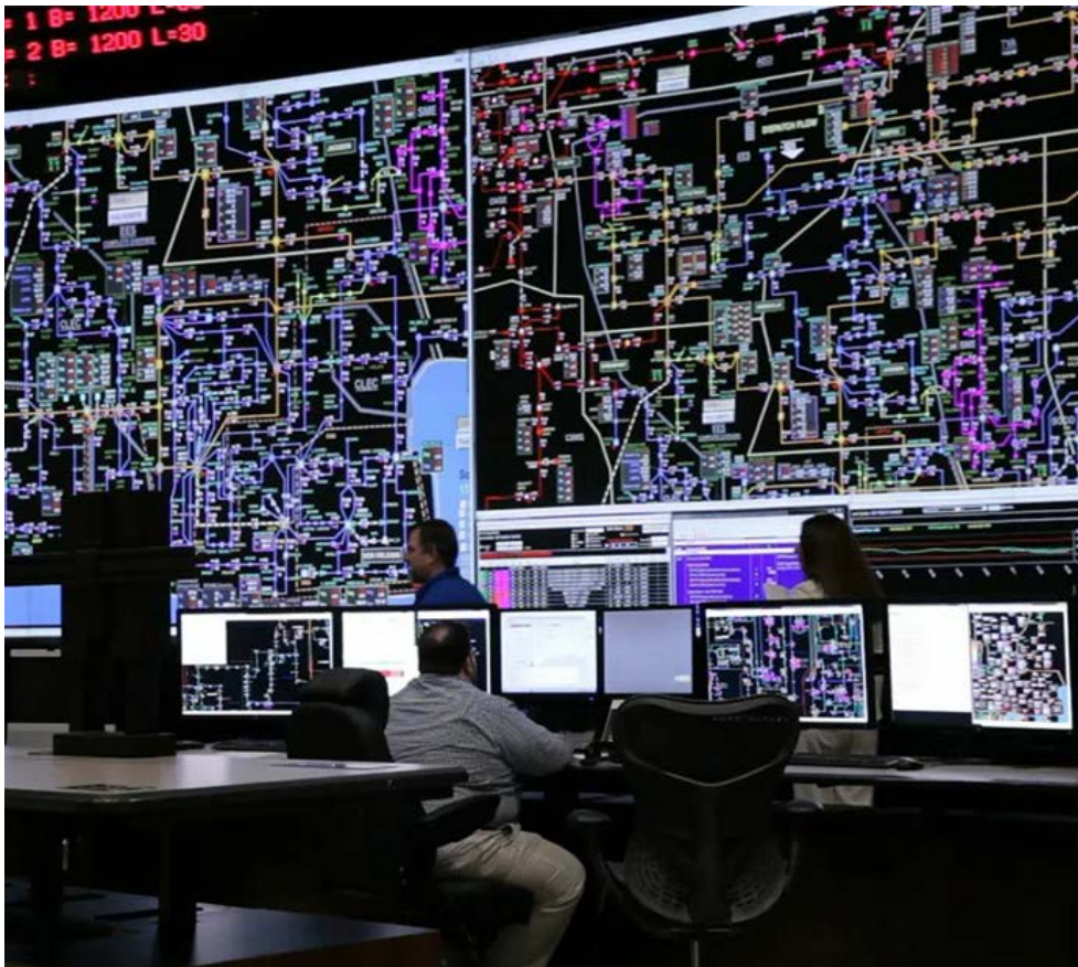
MISO control room | MISO
