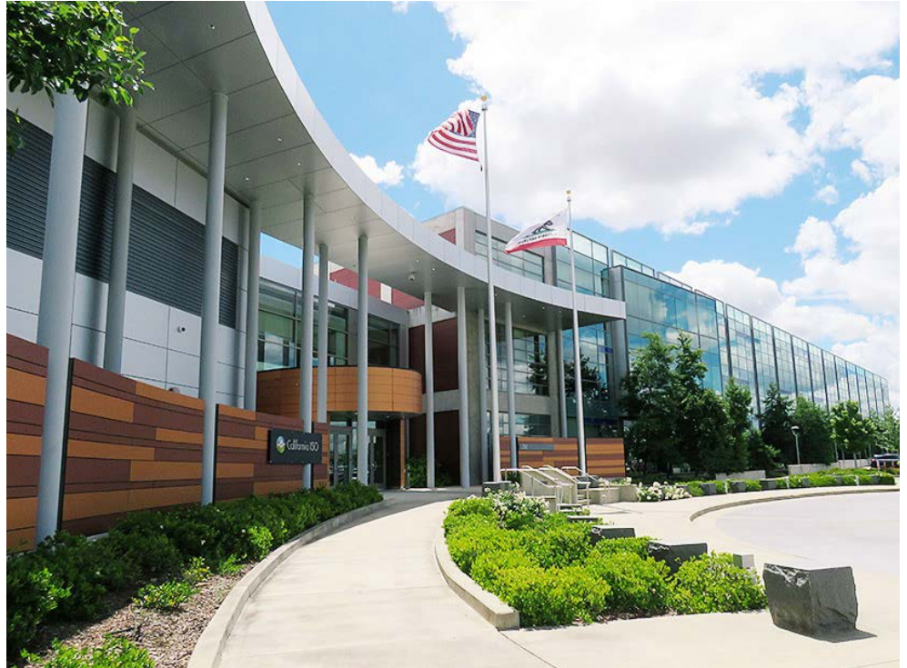
A new proposal calls for the new Western "RO" envisioned by the Pathways Initiative to be based in Folsom, Calif. near CAISO's headquarters for operational reasons. | © RTO Insider LLC
