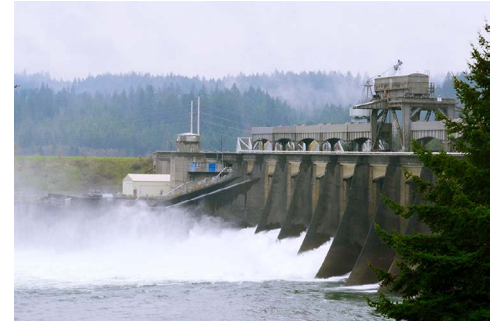
BPA's Bonneville Dam | © RTO Insider LLC
