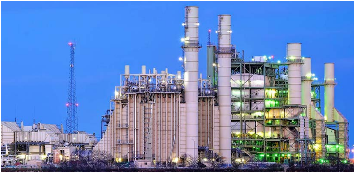
CPS Energy plans to retire three units at its V.H. Braunig facility. | CPS Energy
