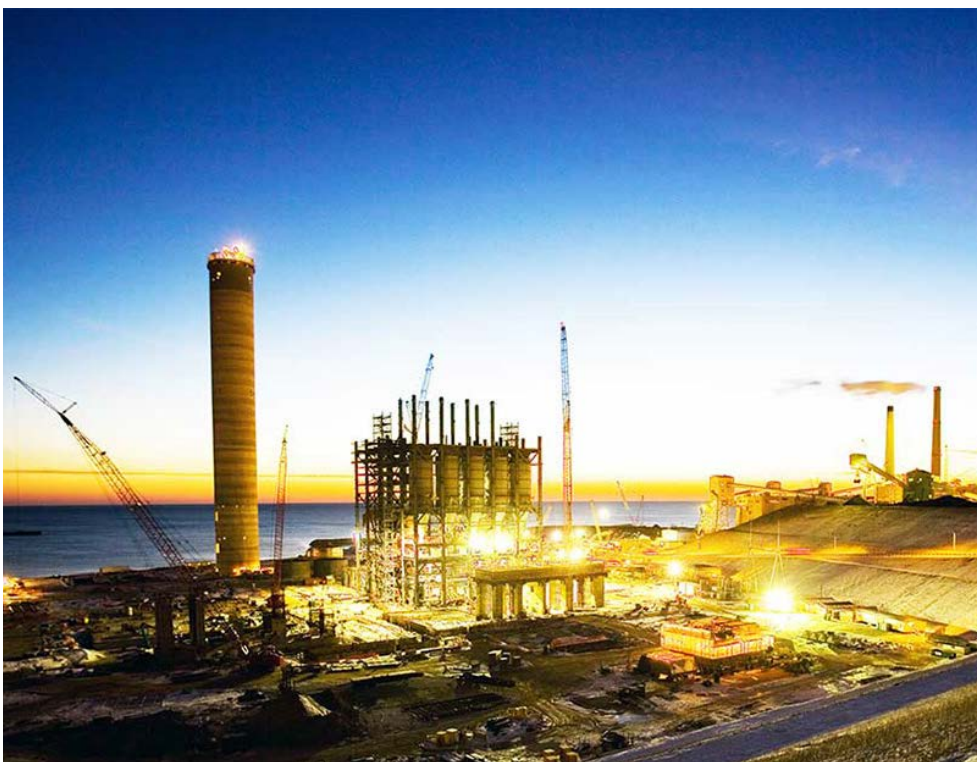
WEC Energy's Oak Creek plant undergoing expansion in the mid-2000s | Bechtel
