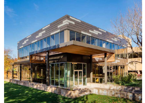
Data centers can come online as quickly as 18 months, potentially adding large loads to the grid, according to WECC. | H5 Data Centers
